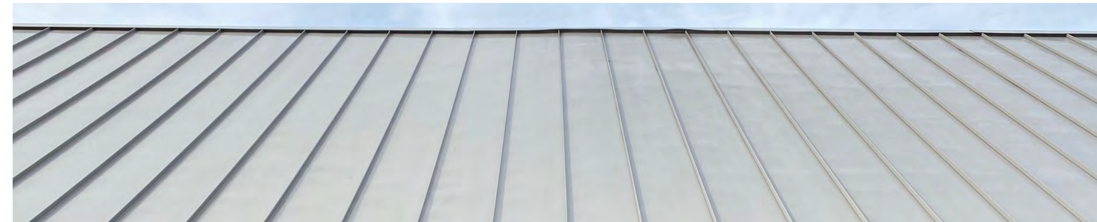
STANDING SEAM METAL ROOF AT NEW ADDITION
