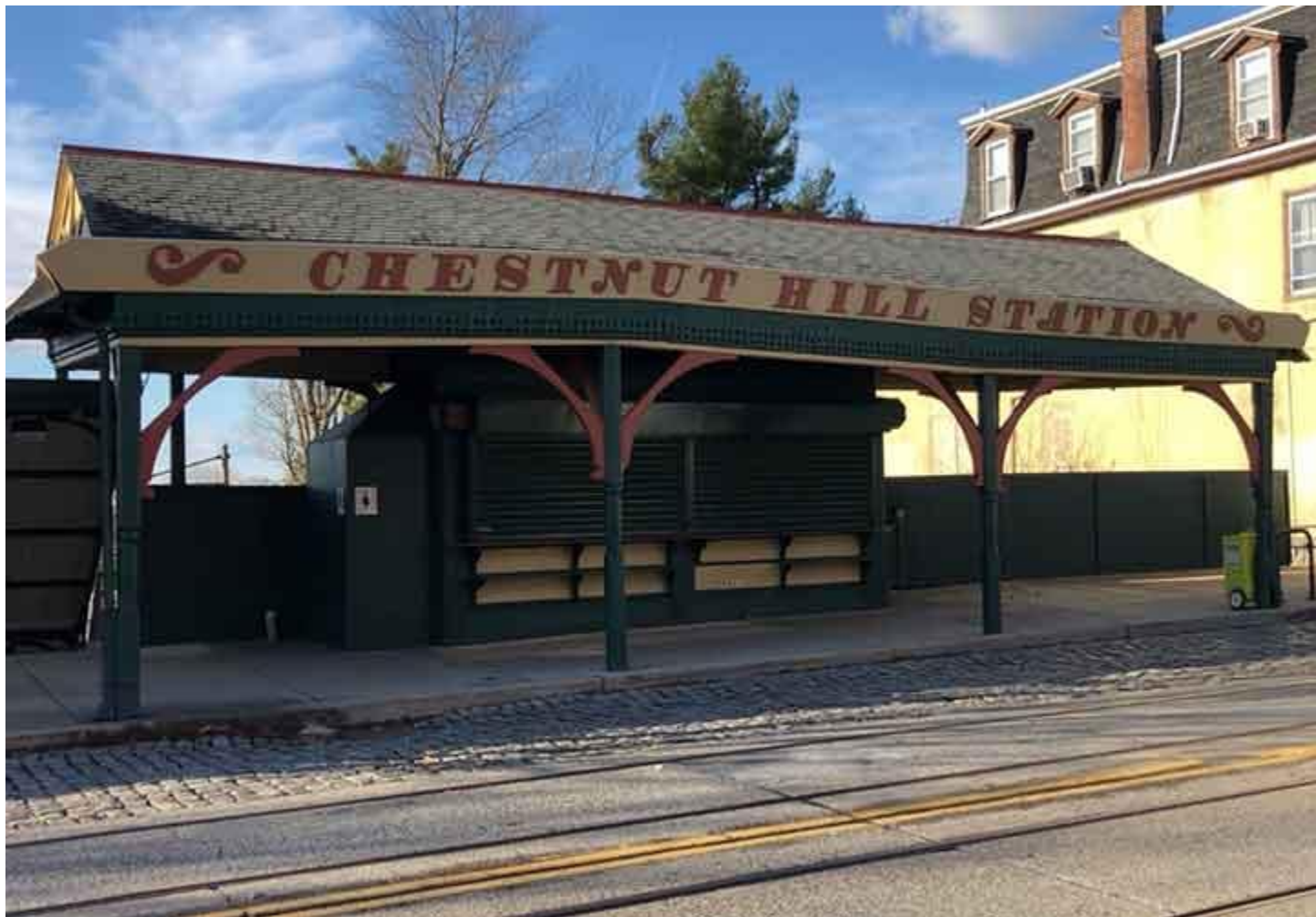
Crews replaced rotted wood, renovated the roof, painted the shelter and performed other structural repairs to the station's canopy. Photo – septa.org
