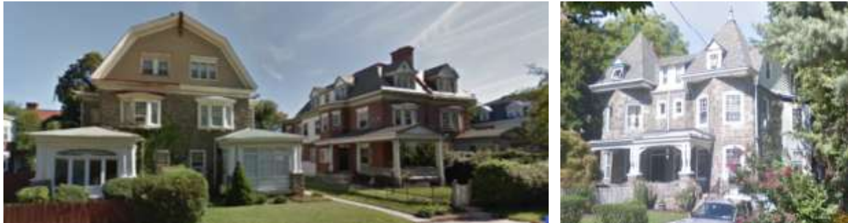
Figure 29. Left: 7000 block of Boyer Street. Right: 100 block E Mt Pleasant Avenue. Source: Google Streetview.
