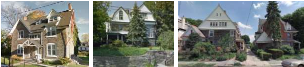
Figure 37. Left: 244 E High Street, rectory for St. Michael's P.E. Church, 1880-81. Center: 221 W Upsal St, dwelling for Jesse A. Tilge, 1887. Right: 108 & 110 and 112 & 114 W. Johnson Street, two sets of paired dwellings, 1887.
