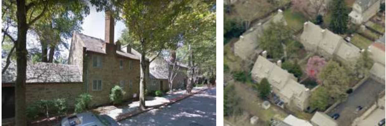
Figure 35. Left: Cotswold Village, 8000 Block of Crefeld Street (1921, Edmund B. Gilchrist), Right: Roanoke Court, 8014-28 Roanoke Street (1931, H. Louis Duhring). George Woodward’s Cotswold Village and Roanoke Court were built of rough-cut local stone and topped with steep roofs that recalled the cottages that Woodward had admired during his trips through England’s Cotswold hills.
