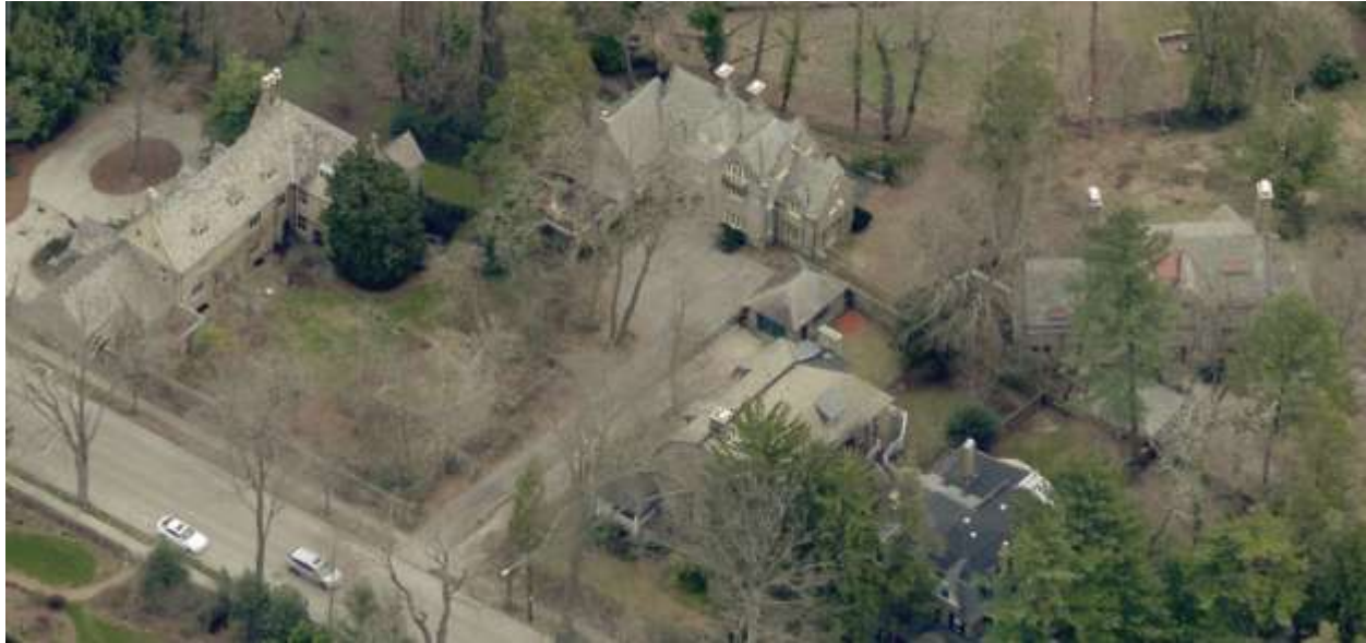
Figure 36. Sulgrave Manor, 200 W Willow Grove Ave (1926, H. Louis Duhring). The Colonial Dames had a replica of George Washington’s ancestral home built for the Sesquicentennial Exhibition held in Philadelphia in 1926. After the Exhibition, Woodward had it dismantled and reassembled in Chestnut Hill, renting it to Robert McLean, publisher of the Philadelphia Evening Bulletin for many years.
