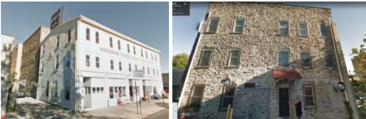
Figure 76. The remaining mill buildings have been repurposed by the Whosoever Gospel Mission & Rescue Home. Source: Google Street View.
