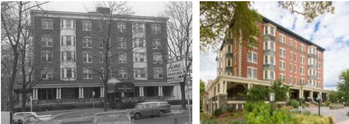
Figure 66. 319 West Cheltenham Avenue, Delmar Apartments. Source: Philadelphia Department of Records (left, 1964); apartmentfinder.com (right).
