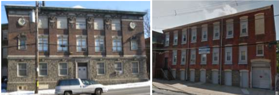
Figure 24. Left: 212-20 Roberts Avenue, Max Levy Autograph. Source: Kim Chantry. Right: 137-45 West Berkley Street, Blaisdell Paper Pencil Company. Source: Google Street View.
