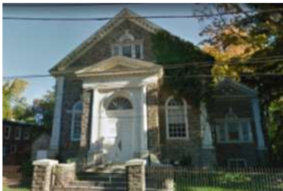
Figure 48. 22 West Penn Street, Trinity Lutheran Church Parish Hall. Source: Google Street View.
