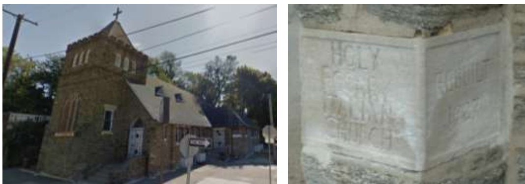
Figure 50. 528 East Haines Street, St. James Methodist Episcopal Church / Holy Rosary Italian Church. Source: Google Street View (left); Pinterest (right).
