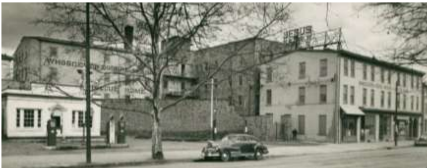
Figure 75. 101 E. Cheltenham Avenue, former mill buildings shown in 1948. Source: Philadelphia Architects and Buildings.
