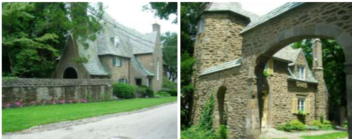
Figure 18. Left: 325 West Allens Lane, also known as Gate House C. Right: 419 Gate Lane. Both properties would contribute to the French Village historic district.
