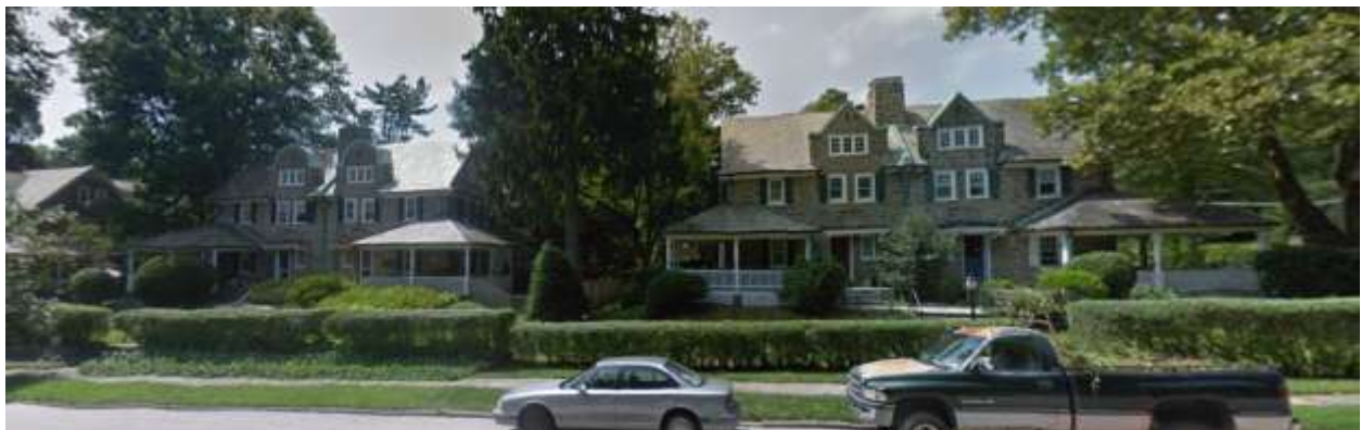
Figure 31. Twin Residences, 7800 block Lincoln Drive (1906, Frank Miles Day)
