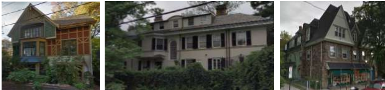
Figure 38. Left: 45 E Penn St, Elizabeth Pearsall Smith house, 1881. Center: 7704-08 Navajo St, Samuel Porcher house, 1908. Right: 8425-27 Germantown Ave, Perseverance Lodge No. 46, Knights of Pythias, 1889.
