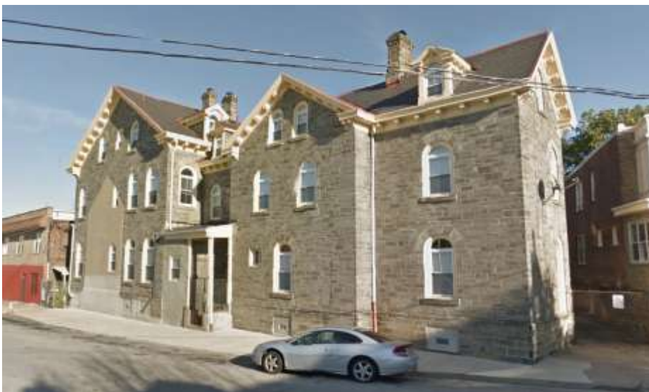
Figure 64. 2 S. Ashmead Street, Heft house. Source: Google Streetview.
